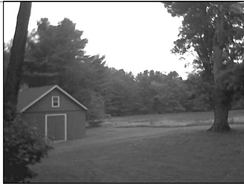
The owners of this homestead are donating a conservation restriction to Kestrel.
